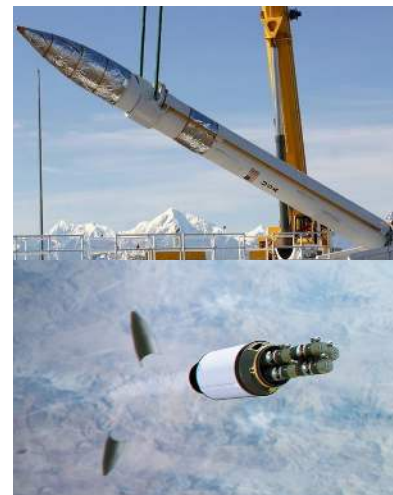
Top: GBI being lowered into its silo
