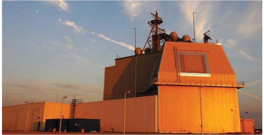
Aegis Ashore Deckhouse Deveselu, Romania
