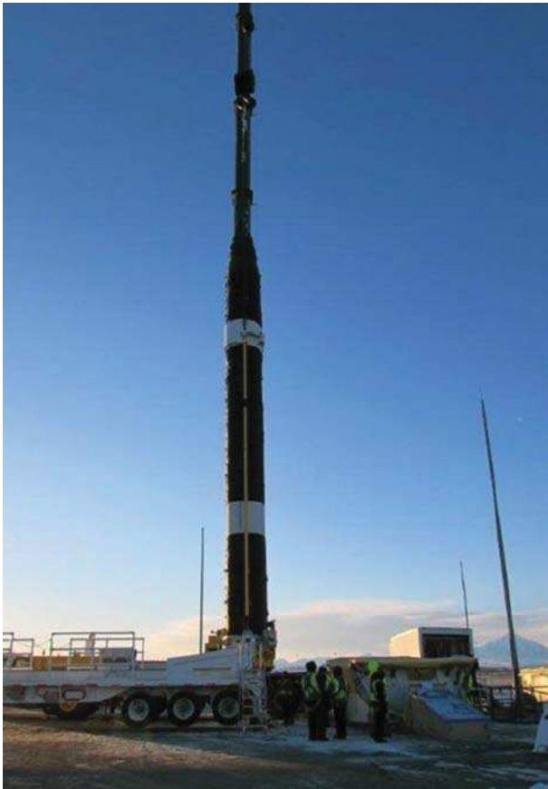
Ground Based Interceptor Emplacement Fort Greely, Alaska
