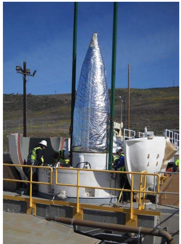
Ground Based Interceptor Emplacement Vandenberg AFB, California
